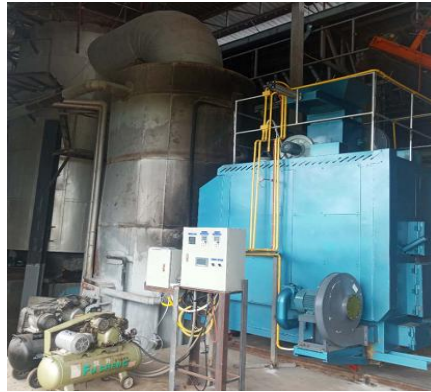
5) 3.0million kcal biomass gasifier connect to 5-ton vertical boiler in Thailand (replace firewood)
