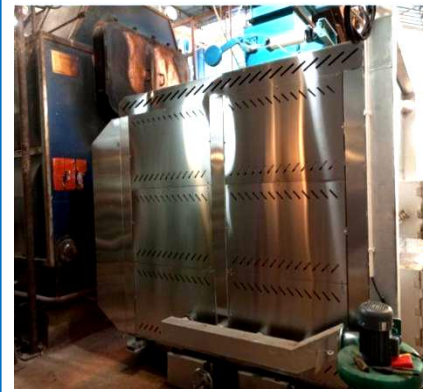
6) 3.6 million kcal biomass gasifier connect to Zhaoqing Xinqiao Food & Beverage Factory's 6-ton hand-fired boiler(replace coal)
