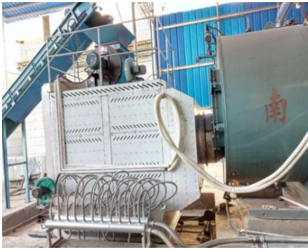
4) 3.6 million kcal biomass gasifier connect to Hengyang glycerin production plant 3500kw thermal oil boiler
